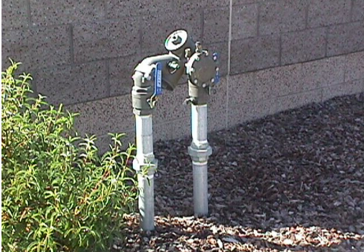
Figure 2. Reduced Pressure Principal Device (RPPD).
