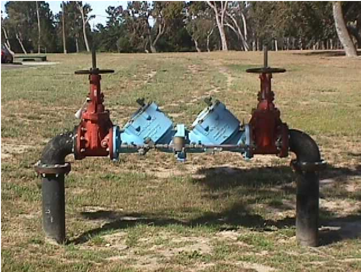
Figure 1. Double Check Valve Assembly (DCVA).
