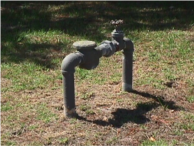
Figure 4. Atmospheric Vacuum Breaker (AVB).
